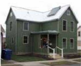
10 Winter Street AFTER weatherization
