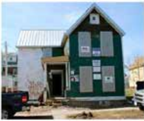
10 Winter Street BEFORE weatherization
