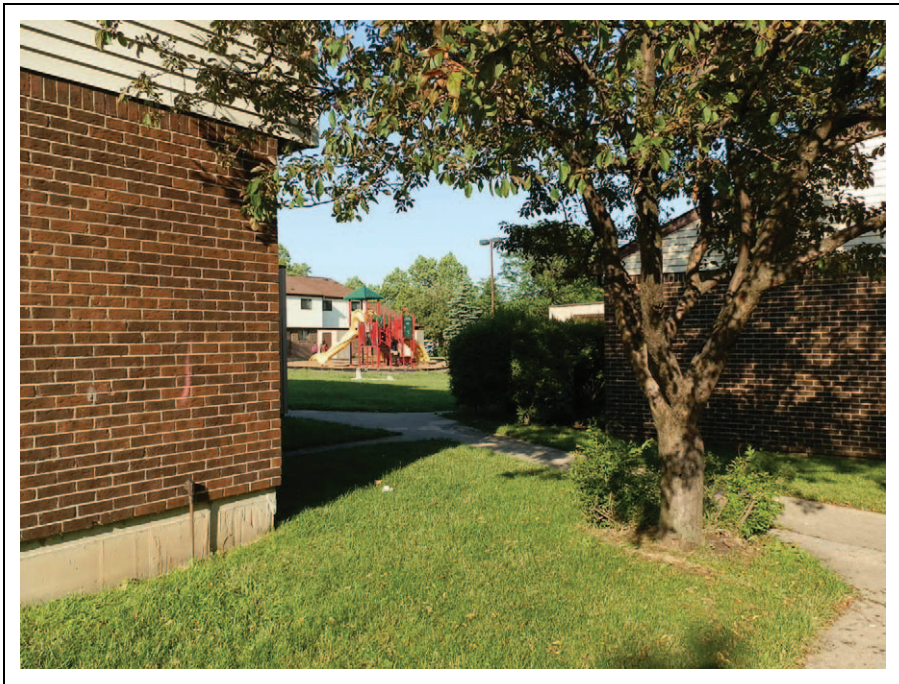
Figure 3. Path leading to the playground in McCarley Gardens.
