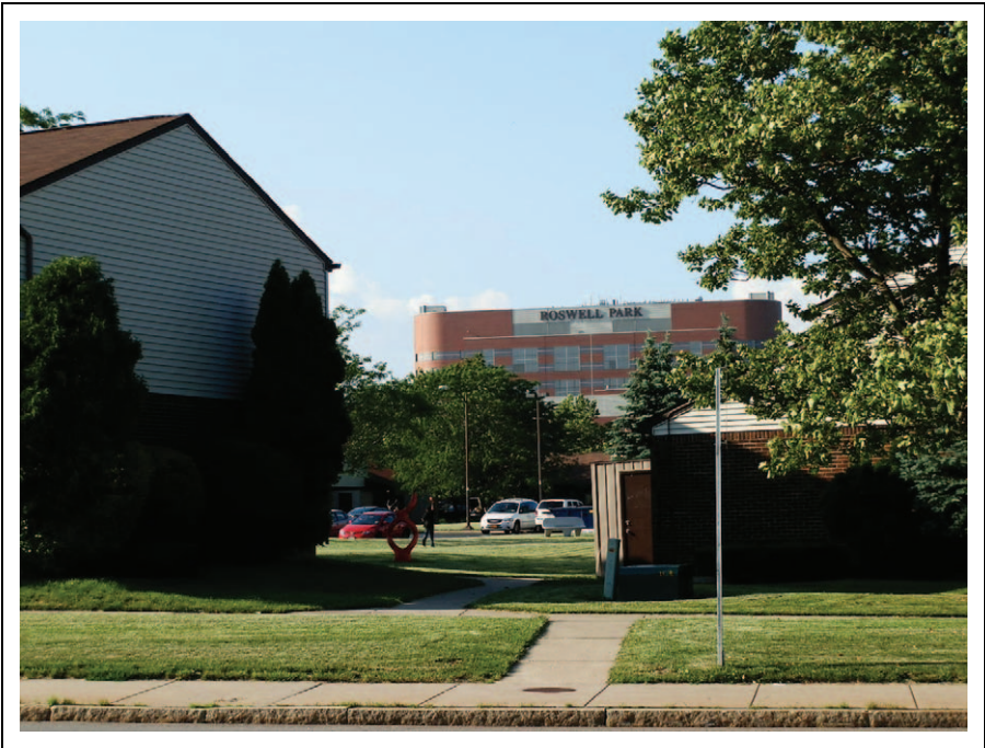
Figure 4. View of Roswell Park Cancer Institute constructed in 1998 from McCarley Gardens.
