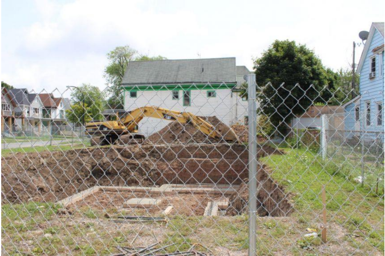
A PUSH development project underway
