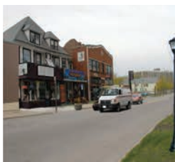
Figure 10 Michigan Street - exist- ing conditions and pos- sible small scale mixed- use development.
