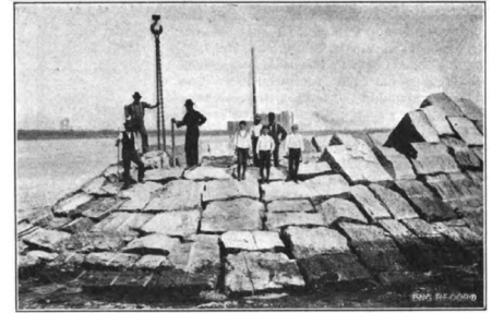
ROUNDING OFF THE END OF THE STONE BREAKWATER.
