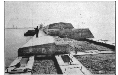
SOUTH HARBOR BREAKWATER, STAGES OF CONSTRUCTION.
