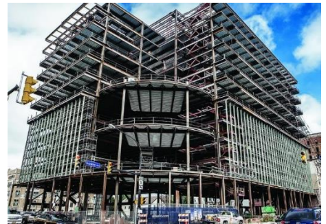
Figure 1. 250 Delaware Avenue Construction.
