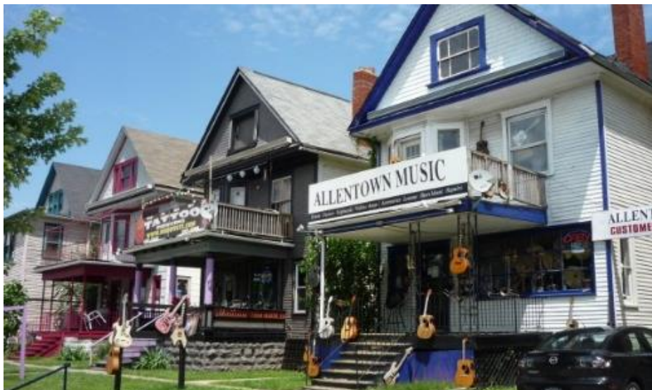
Figure 6. Residential and commercial rental buildings at the corner of Forest and Elmwood Avenue, demolished in 2017.
