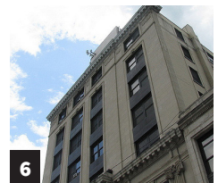
6 Community Bank tower
