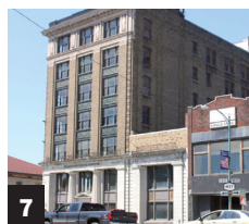
7 Manufacturer's Hanover building
